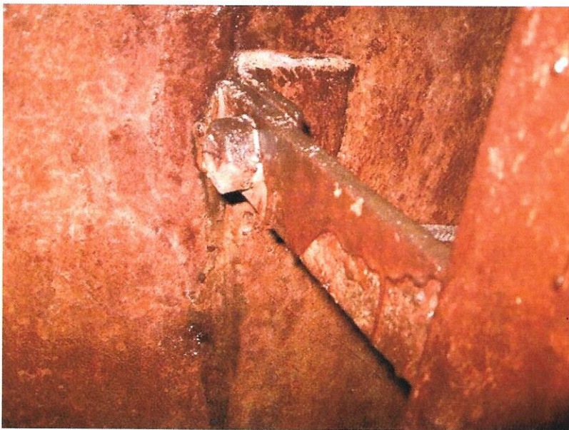
Figure 5. Interior Ladder Anchorage.
