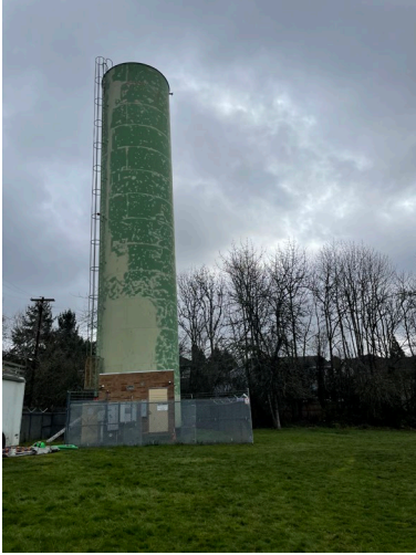
Photo 1: Reservoir and Well Site
