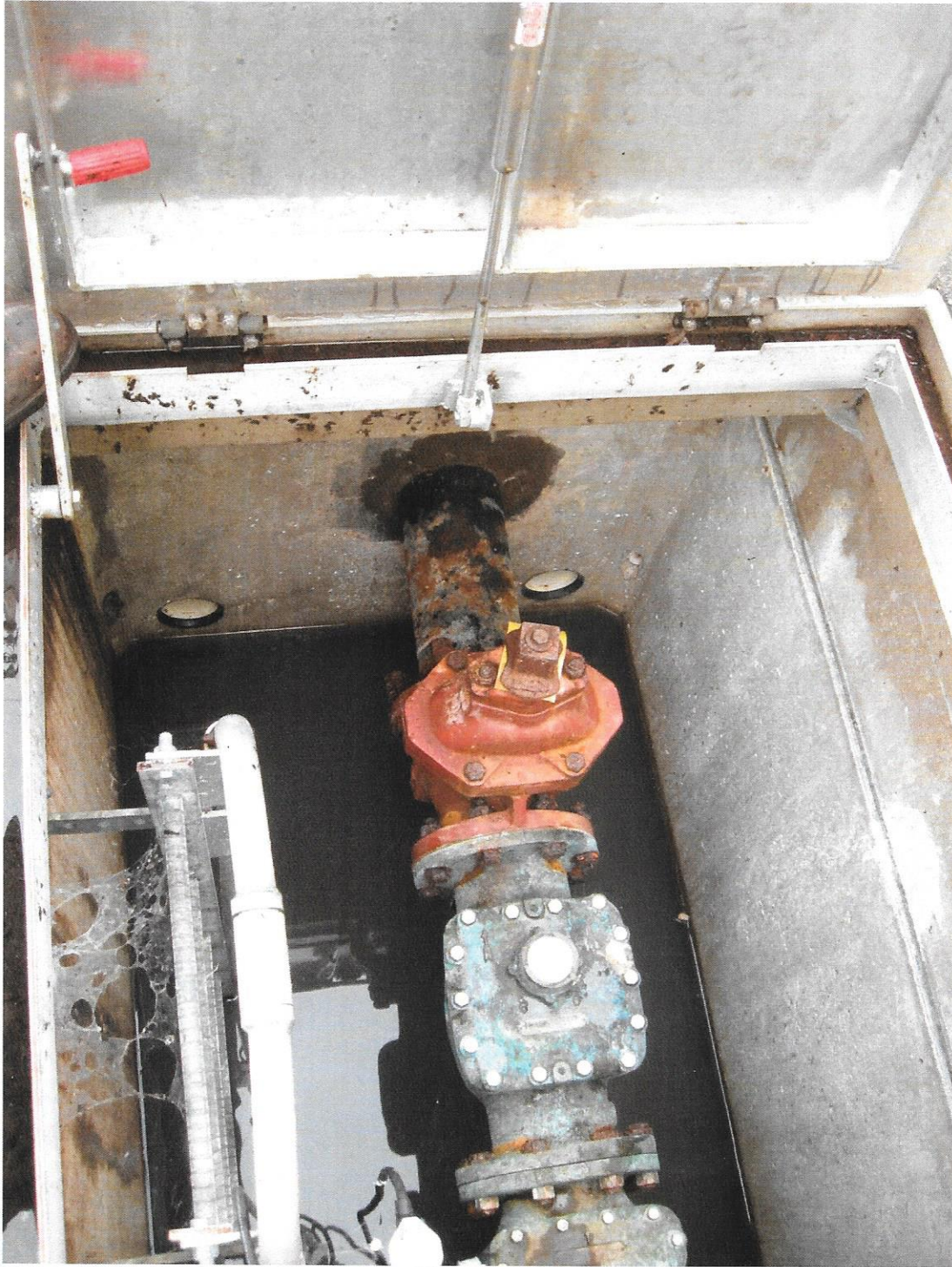
Figure 13. Piping Adjacent to Tank and Pumphouse
