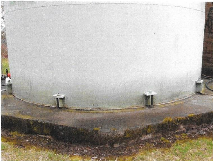
Figure 11. Tank Exterior Anchorage
